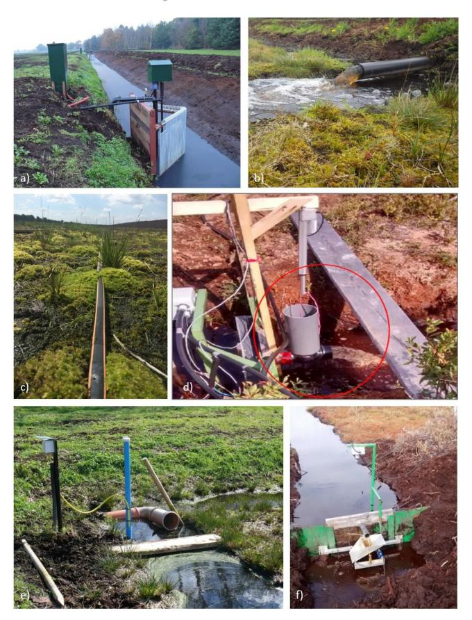
Figure 4. Water management components for Sphagnum farming sites: a) electric pump (Rastede); b) inlet into the irrigation ditches (Rastede); c) drip irrigation (Drenth); d) 'adjustable ditch' with an outlet (Shippagan 2); e) outlet with a data logger (Rastede); f) outlet (Saint-Modeste). Photos: a) and e) Sabine Wichmann, b) Greta Gaudig, c) Dorothea Rammes, d) and f) Peatland Ecology Research Group.
