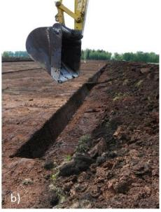
Figure 3. Setting up a Sphagnum farming site on former bog grassland in Germany (Rastede), using an excavator for a) removal of the degraded topsoil and b) construction of causeways and irrigation ditches. Photos: Sabine Wichmann.
